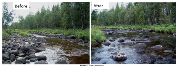
Figure 3. Replacement of stones in streams
