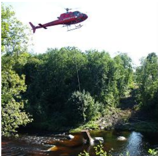
Figure 5. Restoration works involving replacement of spawning substrate by helicopter and excavator (472 tonnes) and large boulders. 486m of shoreline was also restored.
