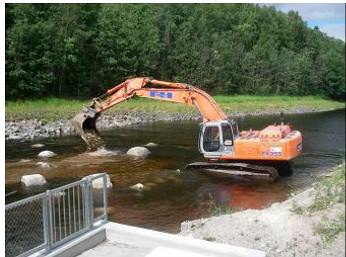
Figure 5. Restoration works involving replacement of spawning substrate by helicopter and excavator (472 tonnes) and large boulders. 486m of shoreline was also restored.
