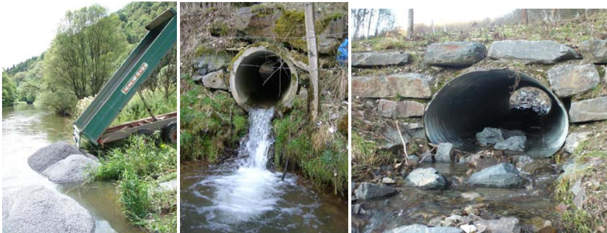
Figure 3. Addition of gravels to main channel and removal of obstacles to host fish migration in tributaries.
