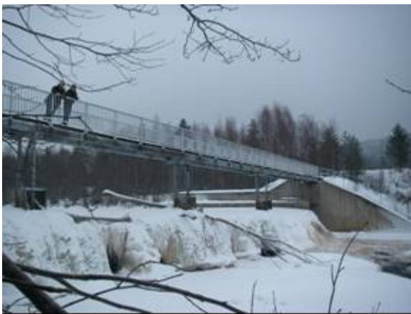
Figure 1. Dam on Nätraån. Left image shows scale of dam (top 42m long and fall 2.3m). Image on right shows non-functional fishway.
