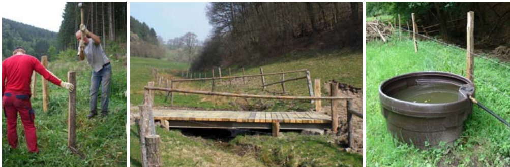
Figure 2. Installation of 2.5km fencing, cattle bridges and watering points.
