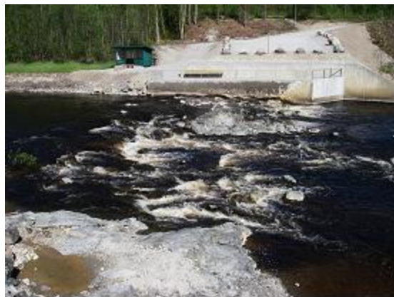
Figure 3. Site post removal of the dam
