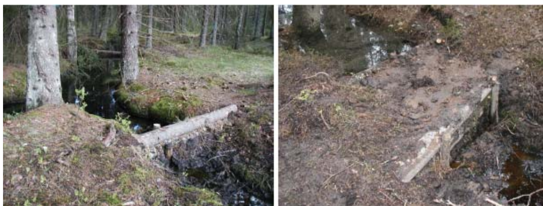
Figure 5. Blocking of ditches to prevent sediment transport.
